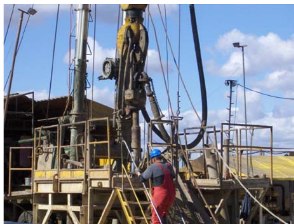
Figure 7: Ongoing drilling project for geothermal exploration in Szentlőrinc MT/gravity survey area.
